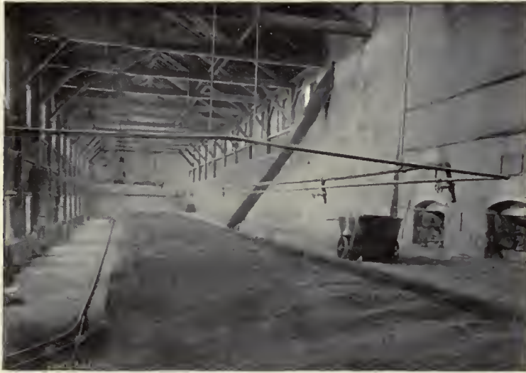
COOLING FLOOR OF BI-METALLIC MINING CO.'S CHLORIDIZING MILL, PHILIPSBURG.
